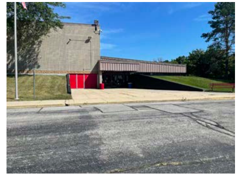
Main Entry to the Building
