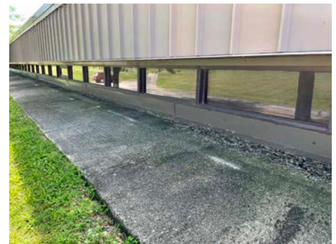
Exterior Clerestory Windows
